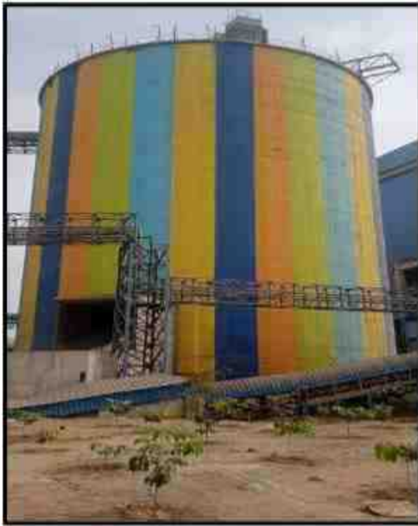
Clinker storage silo
