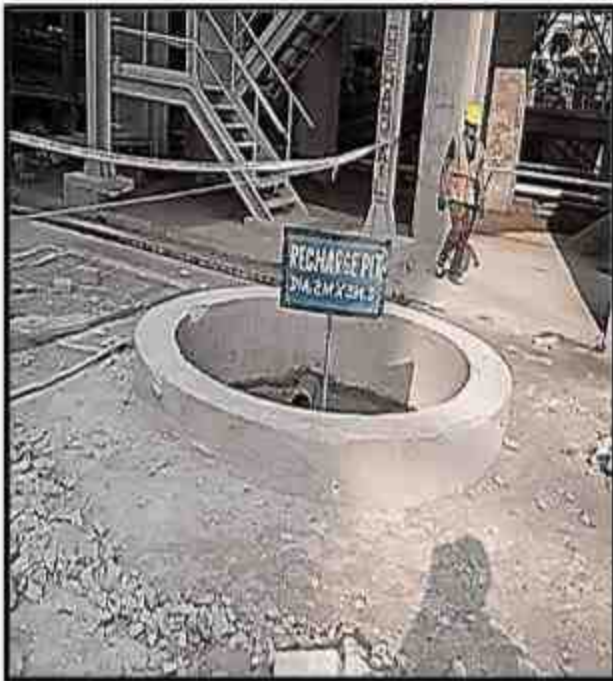
(4) Rain water recharge pit with connecting drain near mill area
