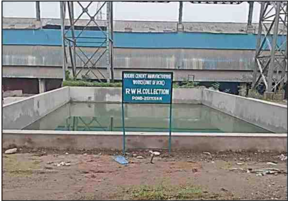
Rain Water collection Pond constructed Capacity: 925 KL
