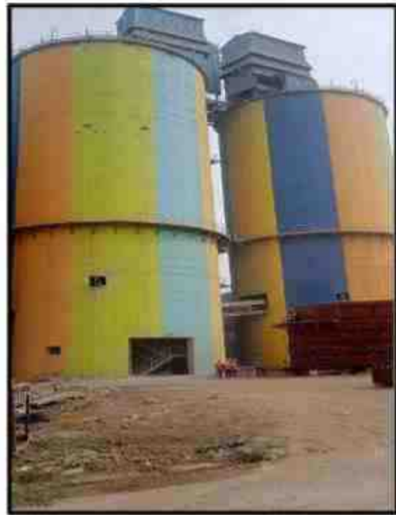
Cement storage Silo
