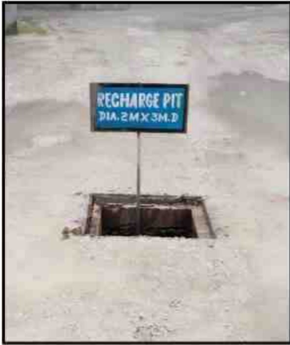
(6) Rain water recharge pit near packing plant covered with chamber and its connecting drainage
