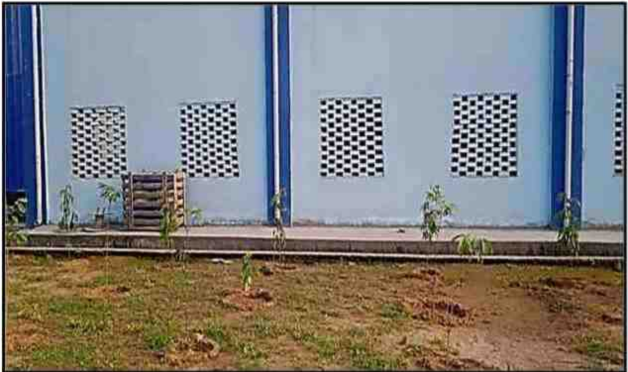
Rooftop Rain water collection pipe line, concreated drain connected to recharge pit near Packing plant building
