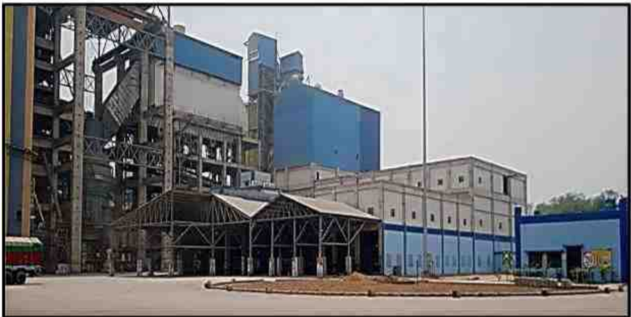
Covered packing plant
