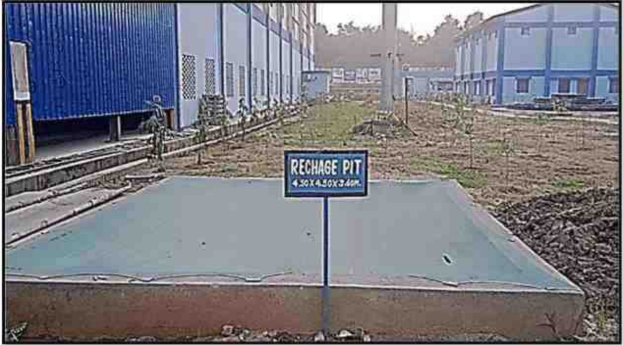
(1) Rain water harvesting recharge pit near Packing plant
