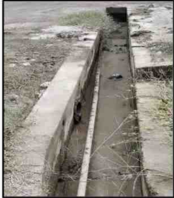
(6) Rain water recharge pit near packing plant covered with chamber and its connecting drainage
